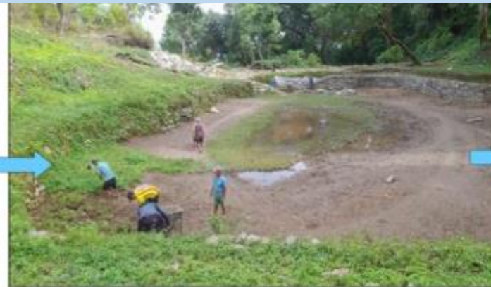
Pond restoration activities (site clearance)
