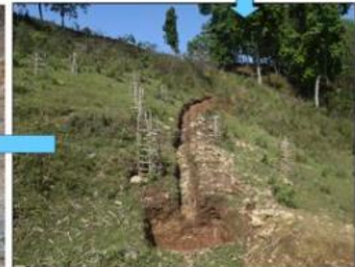
Construction of trenches and siltation chamber
