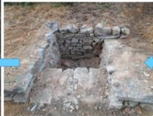
Construction of trenches and siltation chamber
